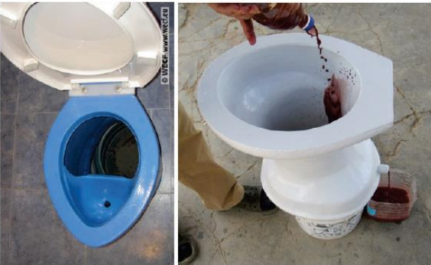
Figure 5. Left: A painted concrete urine diverting pedestal in Bulgaria (photo: WECF, 2007). Right: Ceramic pedestal with an innovative urine diversion concept developed in South Africa and Namibia (photo: Clay House Project, 2011).
