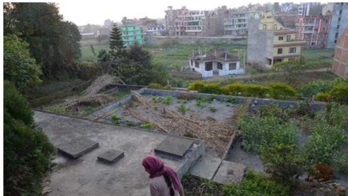
Figure 1.2: Semi-functional constructed wetland for decentralized wastewater treatment in Thimi Municipality, Nepal. Source: D. Spuhler 2015
