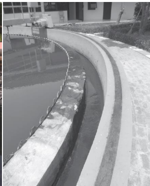
Unbalanced flow from clarifier
