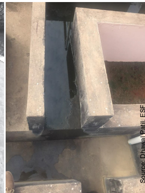
Poor slopes in the channel
