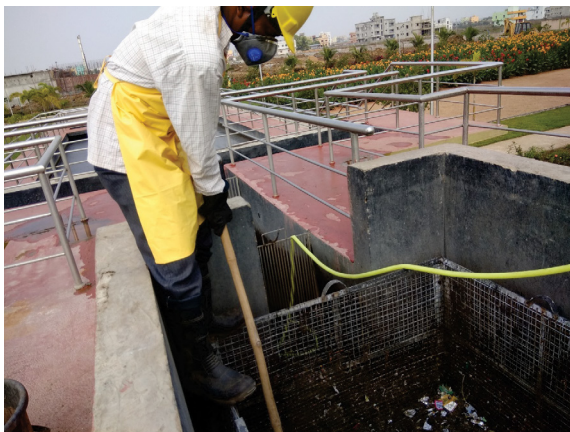
Screen basket without adequate access
