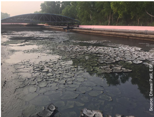
Poor distribution of sludge over drying bed
