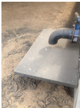
Use of splash plate to reduce erosion and even spreading of sludge
