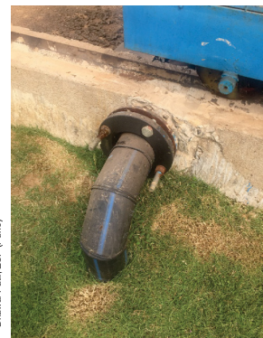
Use of flange joints for easy O&M tasks if needed
