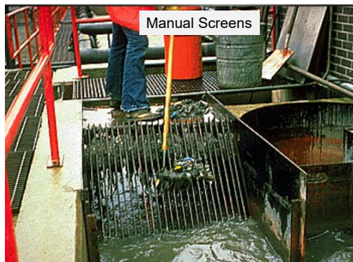
Inclined screens | Perforated tough | Access for operator to rake the screens
