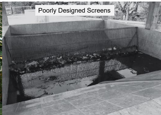
Inclined screens | Perforated tough | Access for operator to rake the screens
