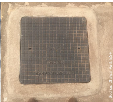
Manhole cover with bituminous coat
