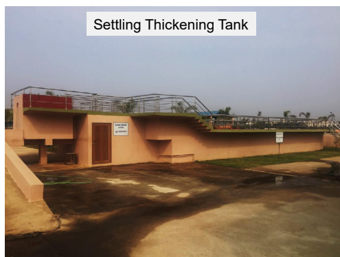
Safety rails | Easy access by road / pathway | Easy access to valves and pipes
