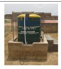
Figure 5. Plastic urine storage tank in Ouagadougou, Burkina Faso installed as part of EU-funded project ECOSAN\_UE, Sept. 2008 (Photo: S. Rüd).
