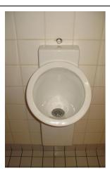
Figure 1. Waterless urinal of Keramag, Germany (model Centaurus). Photo: E. v. Münch.
