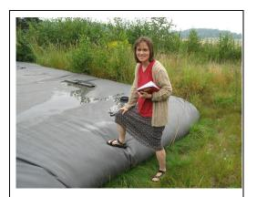
Figure 6. Urine storage tank made of a PVC bladder (3 x 150 m<sup>3</sup>) at Lake Bornsjön near Stockholm (Sweden), Aug. 2007.
